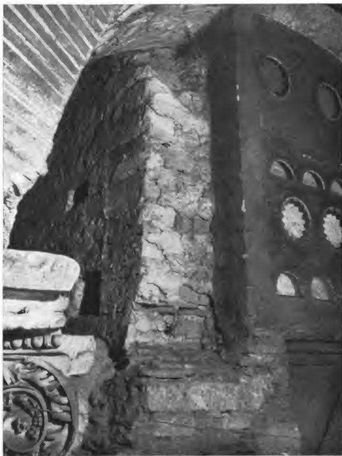
Fig. 226 — S. Maria in Cosmedin. Side wall of the diaconia intersecting the second arch from the left in the Loggia facade (Photo: Corbett).
